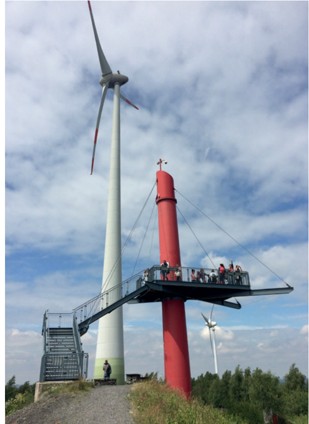
Windmill and overlook structure, Piesberg.
